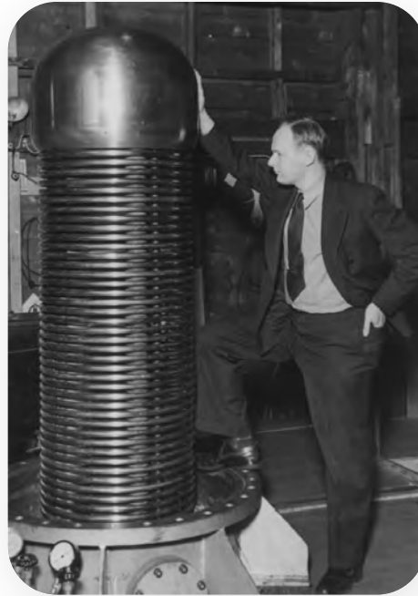
1939: John Trump with a generator
